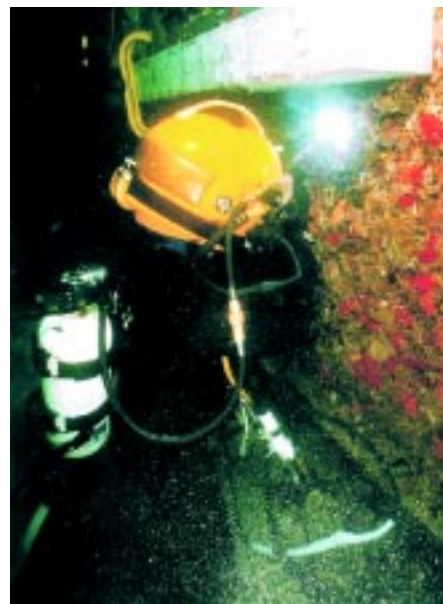
UCT diver conducting wet welds at 120 fsw.
