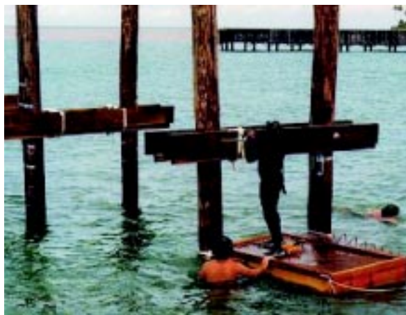
Diver connects pile cap to pile.
